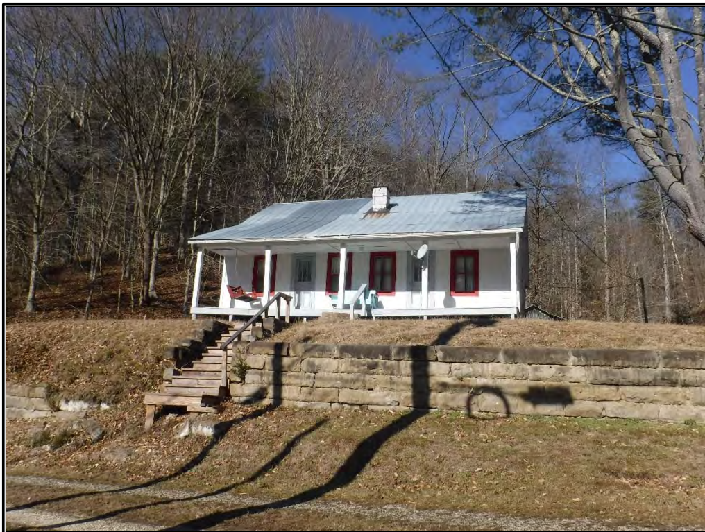
Figure 6. Rock retaining wall and house at north end of project area, facing north.
